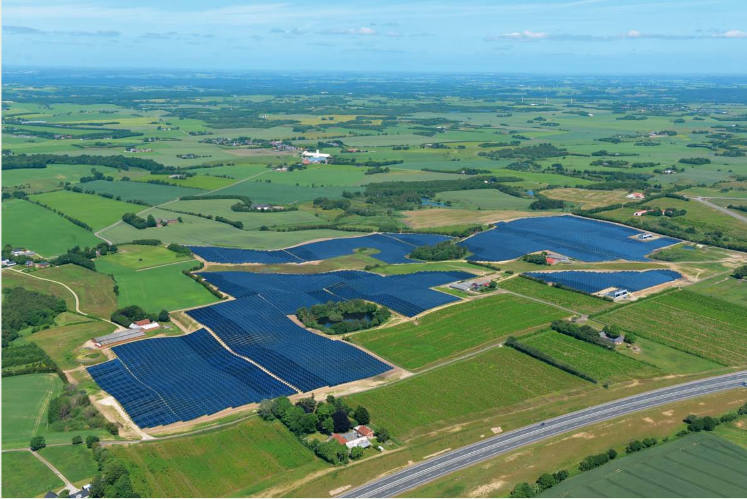
156,694 m 2 solar collector field at Silkeborg, Denmark
